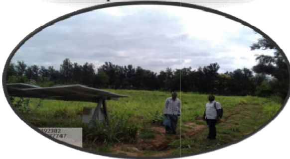
Solar Pump set for irrigation
